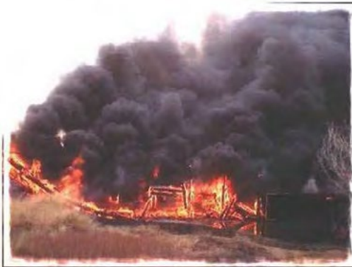
The Bad news: The train stopped with the hot wheel over a wooden bridge with creosote ties and trusses.
