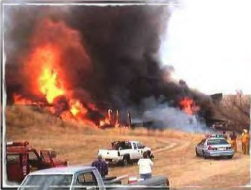
The Bad news: The train stopped with the hot wheel over a wooden bridge with creosote ties and trusses.
