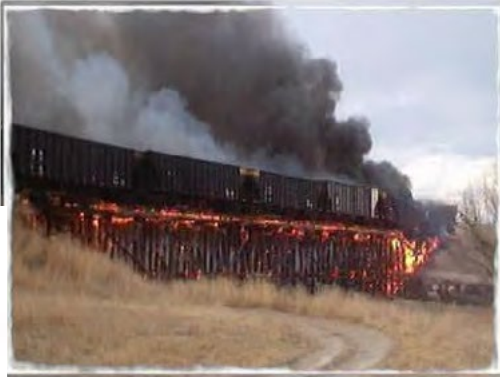
The Bad news: The train stopped with the hot wheel over a wooden bridge with creosote ties and trusses.
